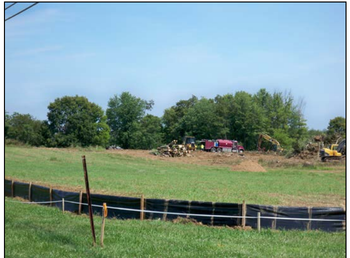
View of Site from end of cul-de-sac
